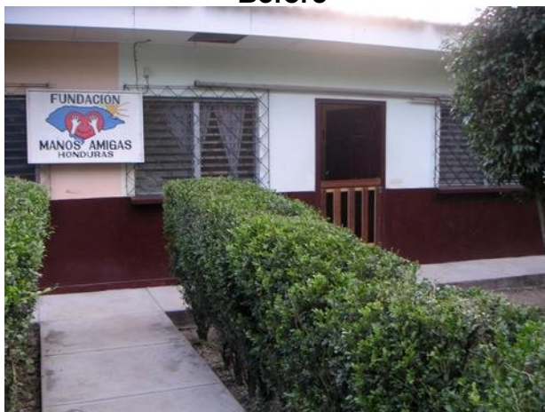
Interim three-room clinic established in 2004
